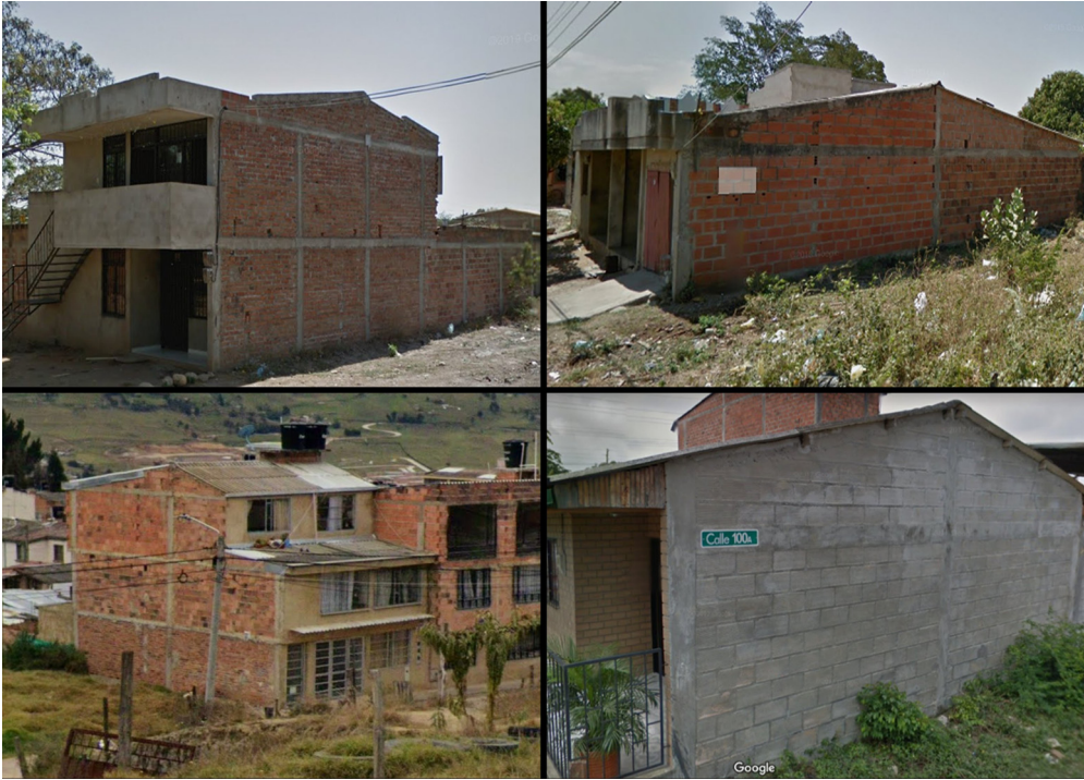
Figure 1. Example of CM houses in Colombia. Images adapted from Google Street View (Google LLC, 2023).
